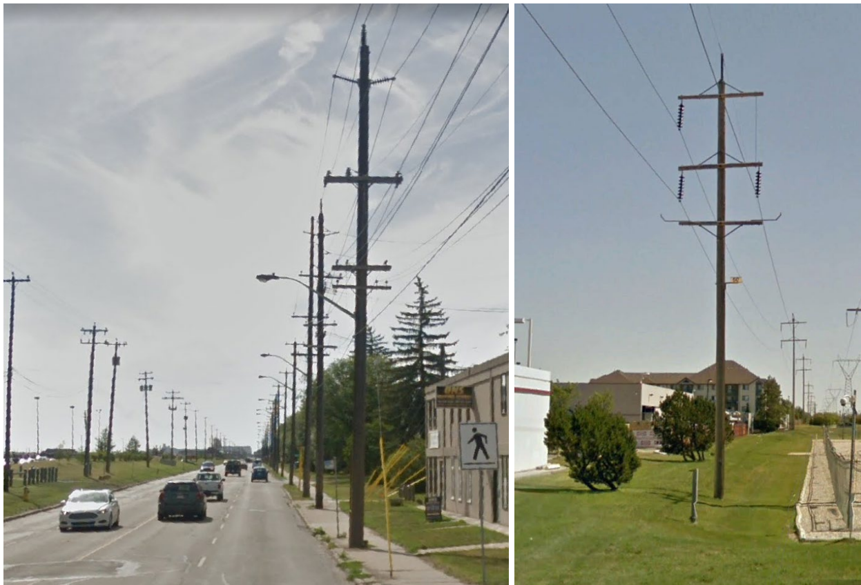
Figure 3 – 72 kV (left) and 138 kV (right) alignment within transportation corridor and URW
